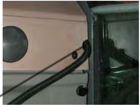
FRONT STEERING CONSOLE - CUT HOLE TO ACCESS POWER SOURCE FOR SWITCH BOX
